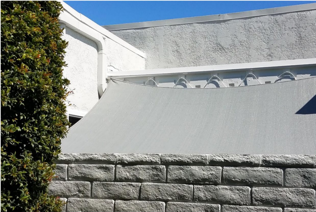
Shade Tarp Attachment to Wall at Window
