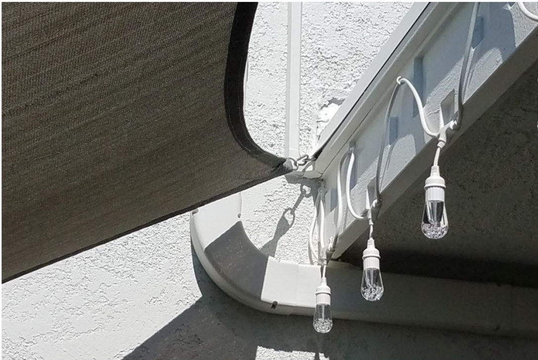
Shade Tarp Attachment to Fascia
