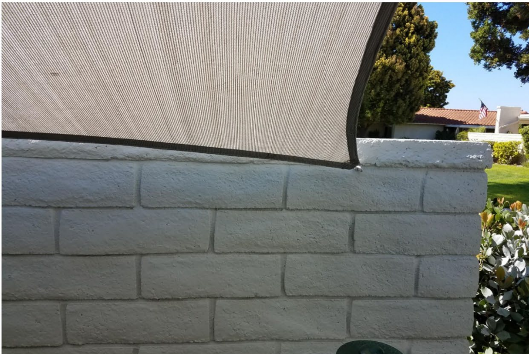
Shade Tarp Attachment to Patio Wall
