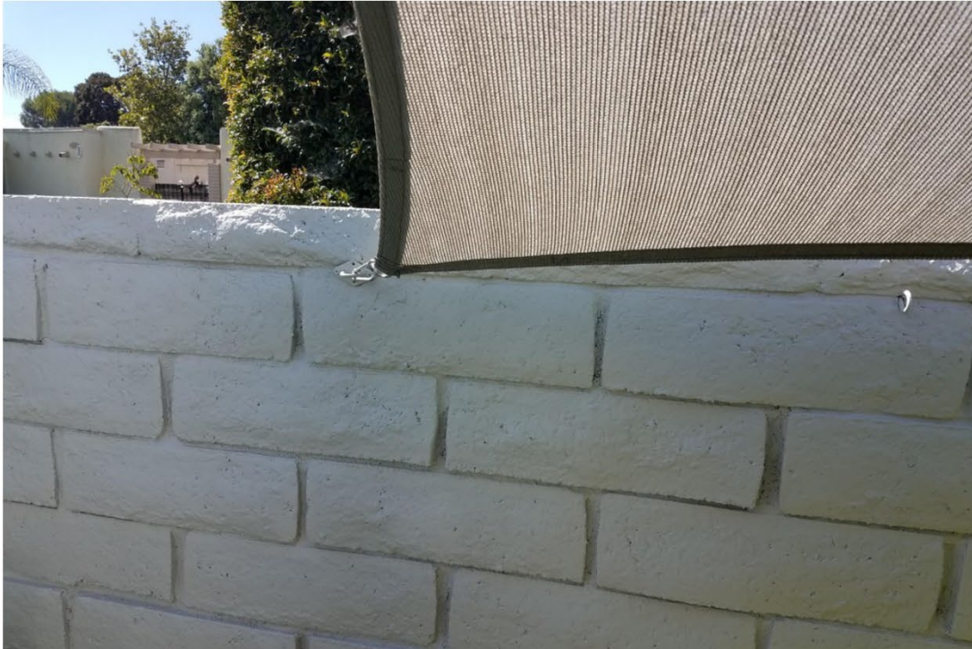
Shade Tarp Attachment to Patio Wall
